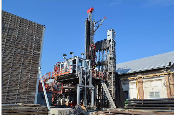
Directional well drilling Photo by InnoGeo Research and Service Ltd.
