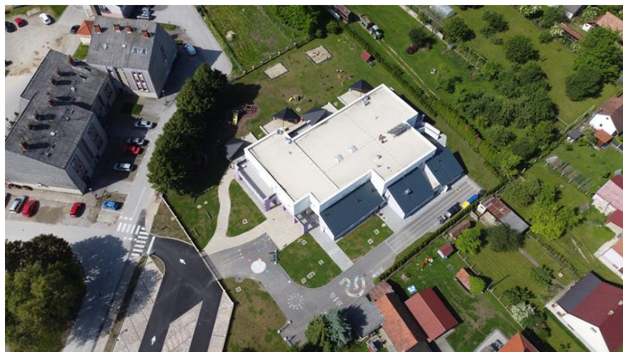
Figure 6.2 Roof area of the Kindergarten "Fijolica" in Prelog
