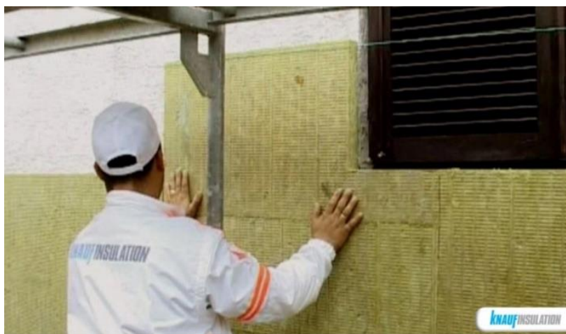
Figure 3. Thermal insulation of exterior wall 3
