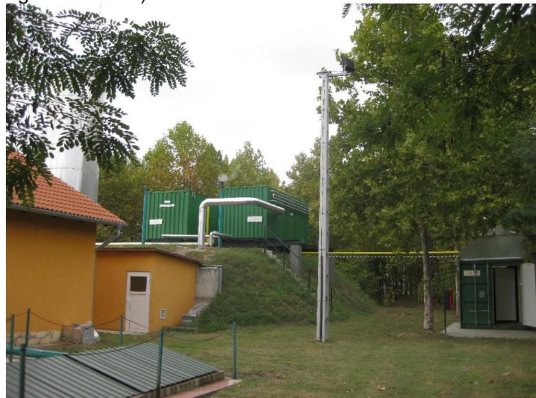
Co-generator prevents atmospheric CH<sub>4</sub> emission and produces enough electric power to run the entire system:
